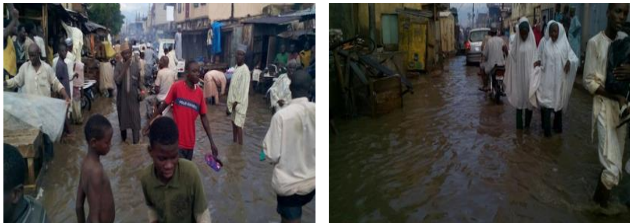
Fig5: Illegal structures and shops built on supposed drainage channels in Kano State resulting in flooding.
