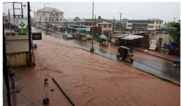
Fig. 7: Poorly designed street roads without drainage system and pedestrian walkway in Anambra State
