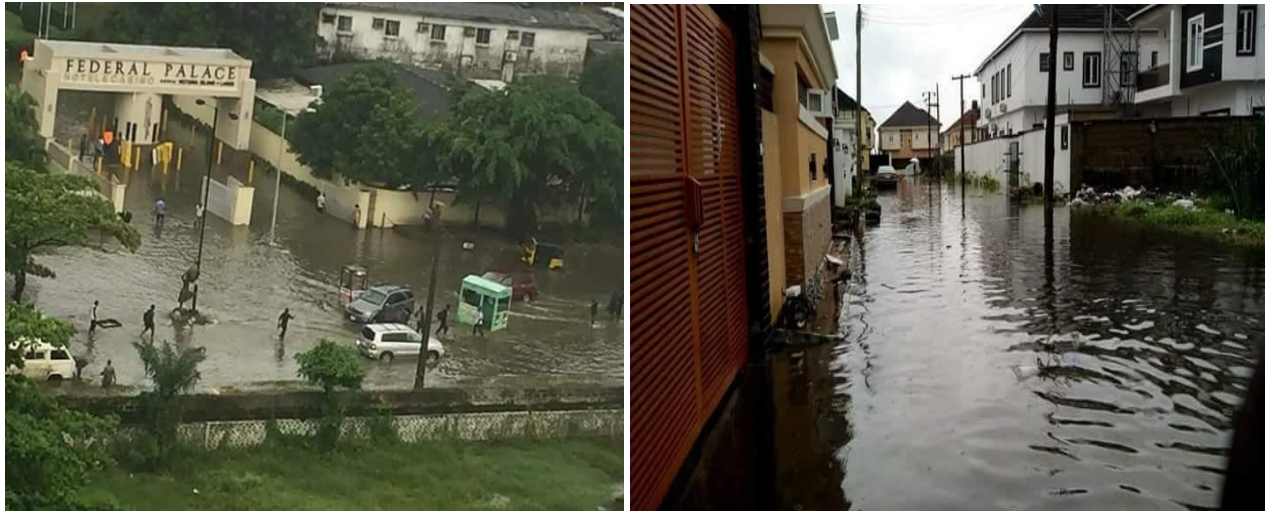
Fig. 4: Flooded beautiful houses built in high-income areas in Lagos state with poor drainage system channels
