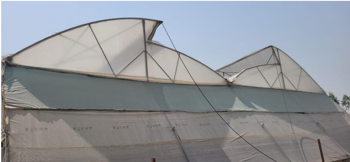
Polyhouse gaseous exchange system (Dev Khara Flowers near KVR hospital Kashipur U.S. Nagar, U.K.)
